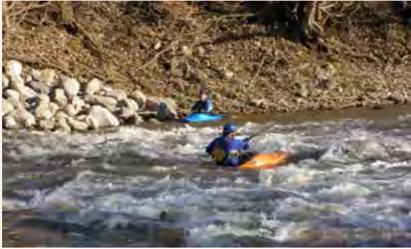
Figure 15 The rock riffle at the Sopers Mill Access was constructed to prevent further erosion and is popular with kayakers and tubers.
