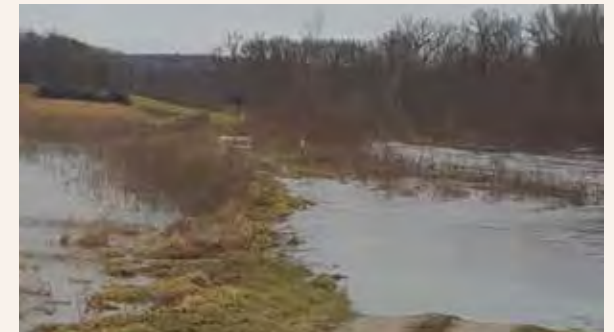
C6.E The adjacent landowner reports water reaches his field during high water through the boat launch at CJ Shrek Access. It appears that when the launch was constructed, the existing elevation of the levee was lowered to accommodate the launch. Resolution of this drainage issue can occur in conjunction with design and construction of an upgraded access.
