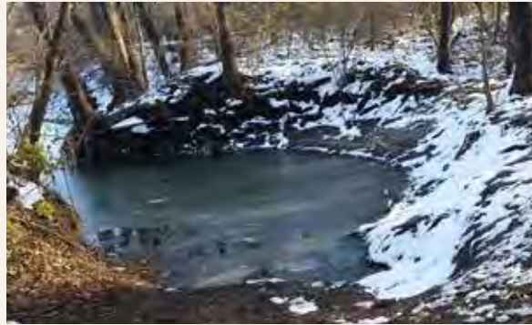
C4.B Erosion at this location is exacerbated by pressure on the streambank from the channel and outflow from Peterson Ponds.
