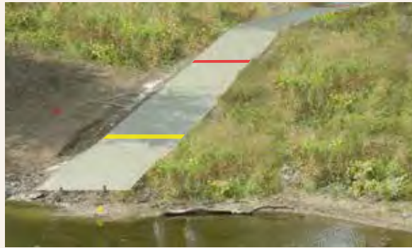
R1.F Physical marking of key flow levels for paddlers at the most popular accesses is recommended. These include the lowest suggested flow and the caution/high flow levels. This graphic illustrate the recommended method to communicate this information.
