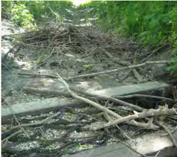
Figure 27 Upgrades at Askew Bridge Access include a hard-surfaced carrydown launch to replace the existing stairs.
