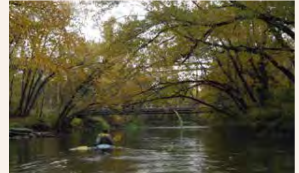
C2.A The City of Story City is interested in refurbishing this dam, seen ahead in this photo. Rock structures designed to mitigate the dam have failed twice due to high water. Retrofit of this dam will leave only one dam on the South Skunk in place - the Hannum's Mill Dam near Ames.
