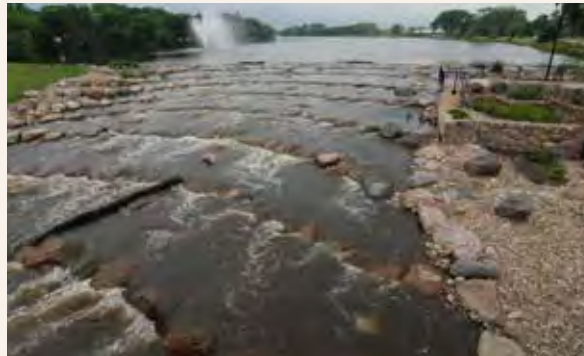
C5.B Rock arch rapids utilized for dam modifications such as the 13th Street Dam enhance the value of fishing on the river.
