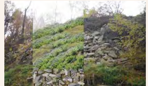
C2.D Following removal of surface debris, revegetation with native shrubs and herbaceous plants is recommended similar to this illustration.
