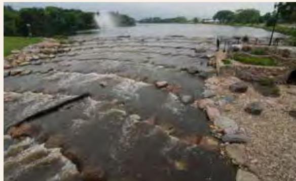
C4.C A series of rock arch rapids are commonly used in Iowa and Minnesota to remove the roller-motion created by low head dams.
