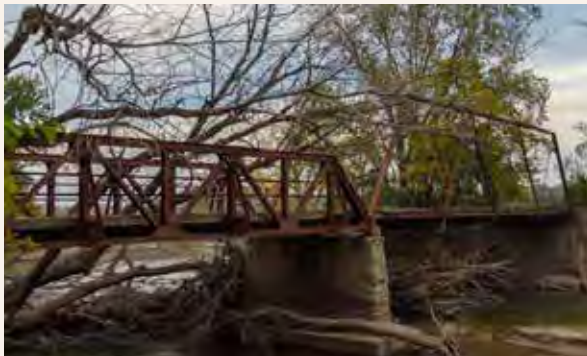
C6.D The historic bridge (right) has been abandoned for many years and is beginning to collapse due to lateral channel migration, causing large-scale streambank collapse near the historic bridge. Large woody debris accumulates near the bridge (right), exacerbating high water damage.
