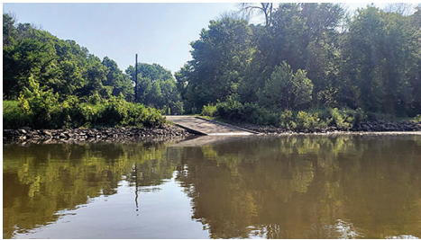
Looking downstream at the George Wyth State Park boat ramp, river left
