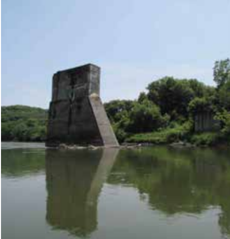
Railroad bridge pilings
